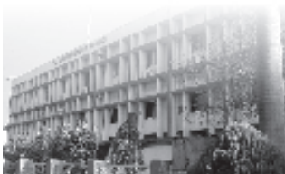
Corporate Office & Works (J-7, Hingna, MIDC)
